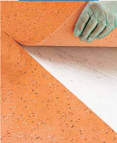
Installation of PVC with Adesilex G20
